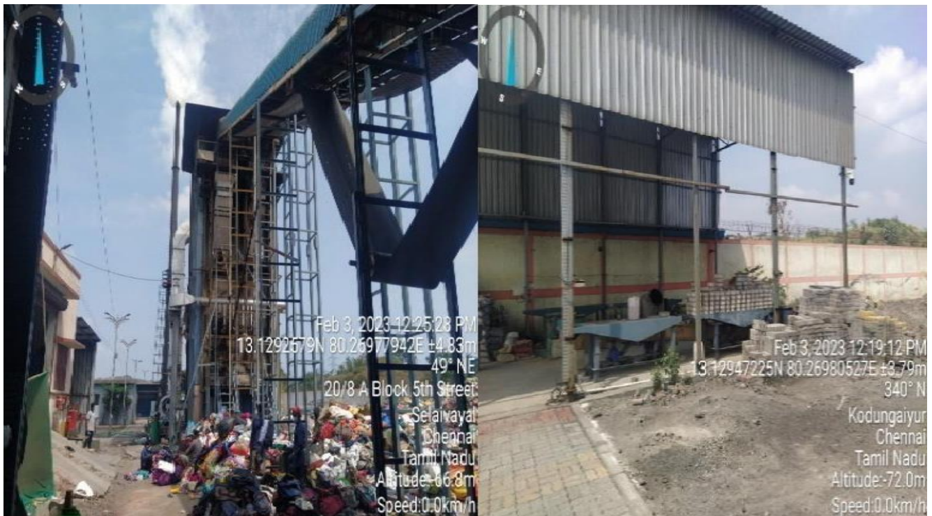
Fig. 8 Incinerator Plant at Kodungaiyur Disposal Ground
