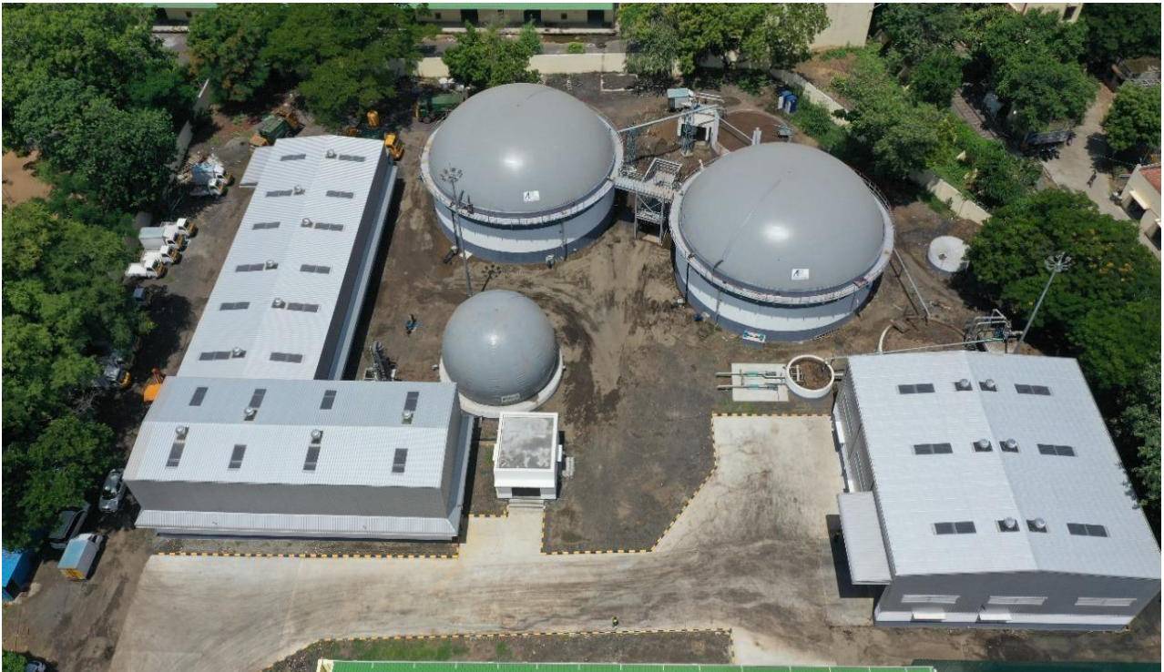
Fig. 9 Overview of SWMS BIO-CNG plant
