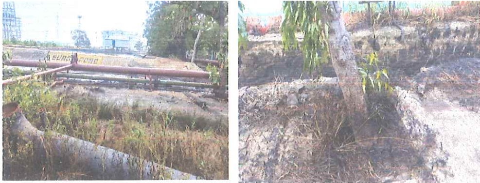
Surge pond and drain opposite to surge pond
