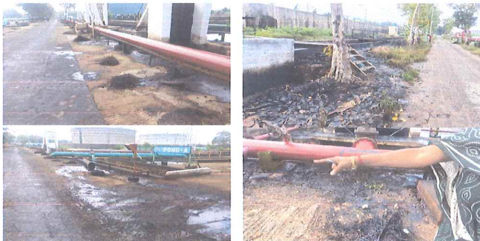
Oil spill observed around Storm water collection Pond A
