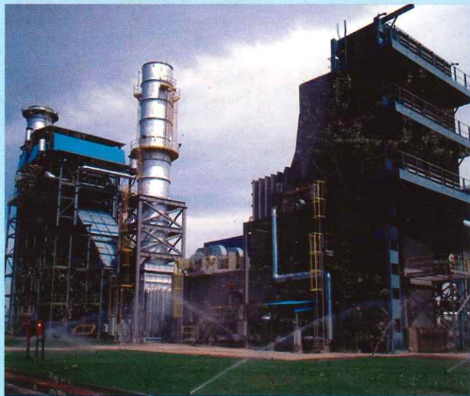
VIEW OF THE POWER PLANT
