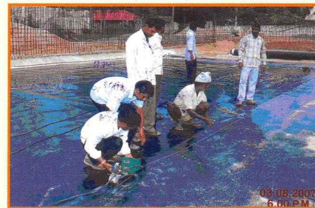
SLF UNDER CONSTRUCTION
