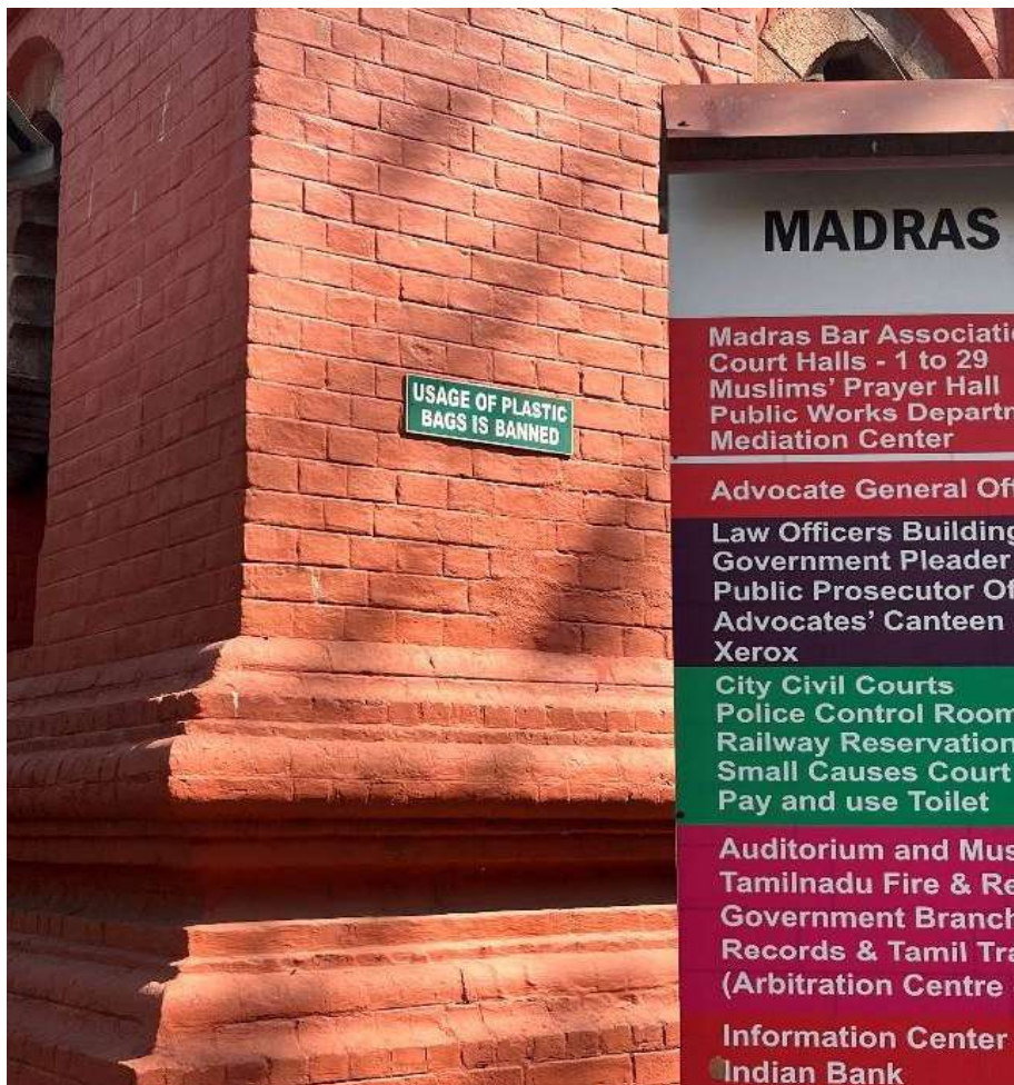
Figure 16. Signage hidden by a bigger board
