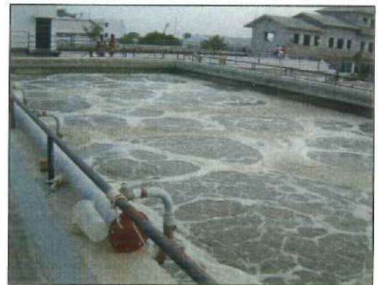
Fig. 3.4 Bio-enzyme Process for Organics Removal
