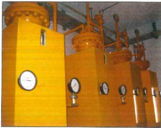
Fig. 4.9 Chlorine Evaporator
