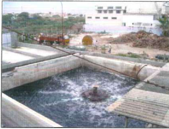
Fig.3.5 ASP for Organics Removal
