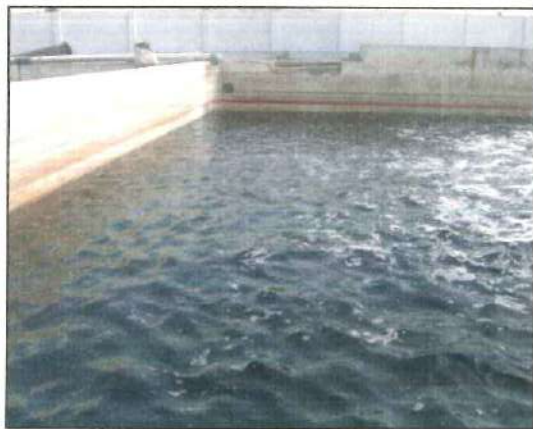
Fig. 4.15 Collection/ Equalization Tank as Chlorine Reactor
