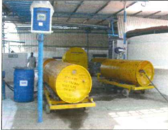
Fig. 4.1 Chlorine Tonners
