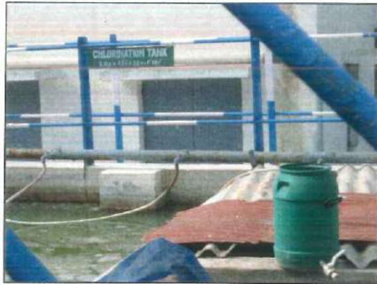
Fig.3.1 Collection Tank as Chlorine Reaction Tank
