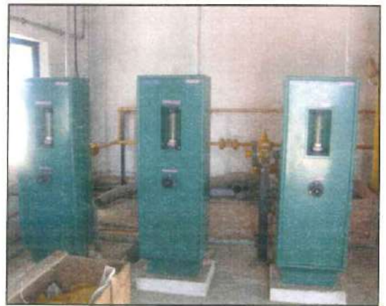
Fig. 4.8 Cabinet Housing for Rotometer
