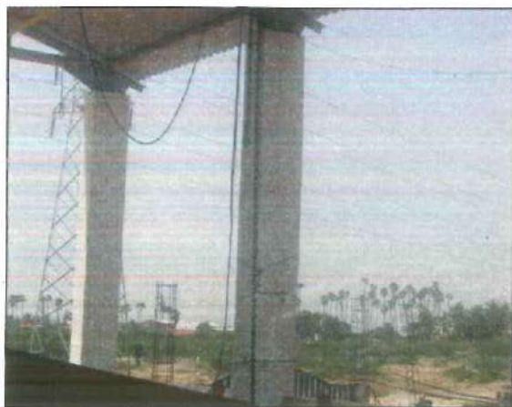
Fig. 4.21 Electric Hoist Cranes
