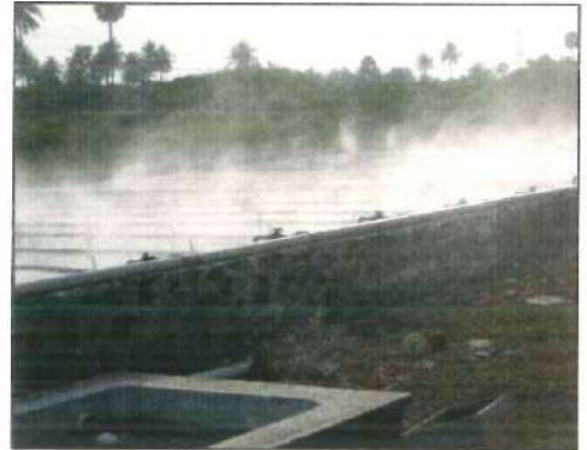
Fig.3.10 Enhanced Solar Evaporation Pond
