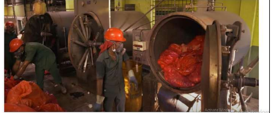
Loading of Red category waste to Autoclave
