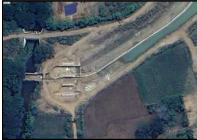
Fig No 1.3 Diversion of Narimudukku Drain into existing south rajan channel by constructing baffle wall at the centre of channel
