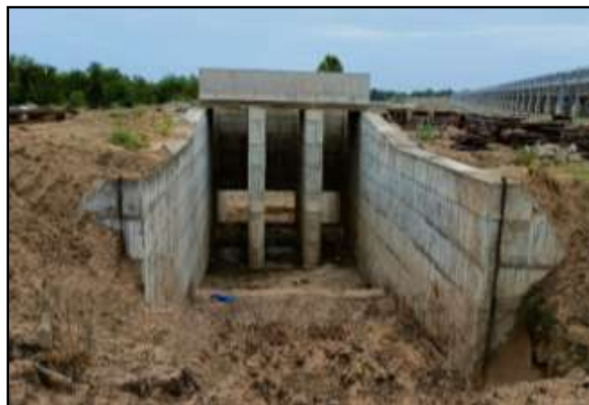
Fig No 1.2 Head sluice of south rajan channel
