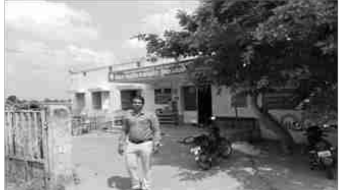
PRIMARY HEALTH CENTRE-POIYATHANALLUR VILLAGAE
