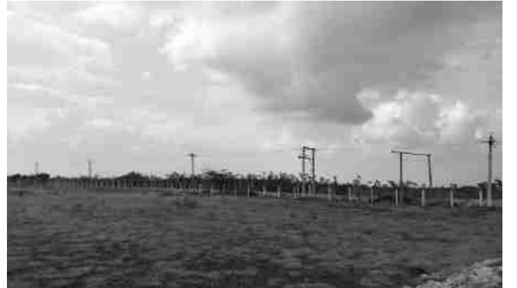
6. Power Line – 50m (NE-SW)
