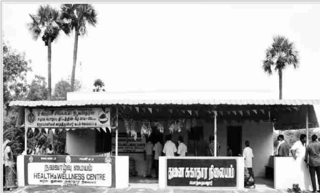
CONSTRUCTION OF WAITING HALL IN HEALTH AND WELLNESS CENTER IN MOTHAIYANUR VILLAGE – Rs.3 LAKHS
