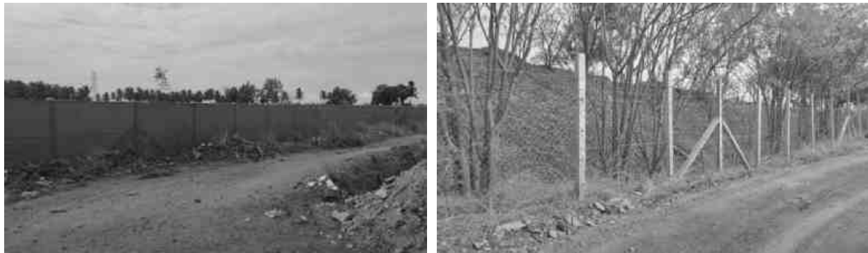
Fencing at Project site
