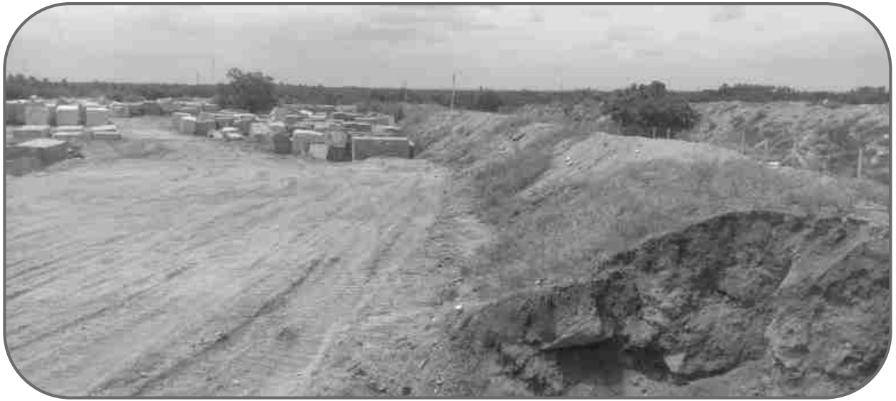
FIGURE 2.1A: FENCING AND SOIL BUND OF THE PROJECT AREA
