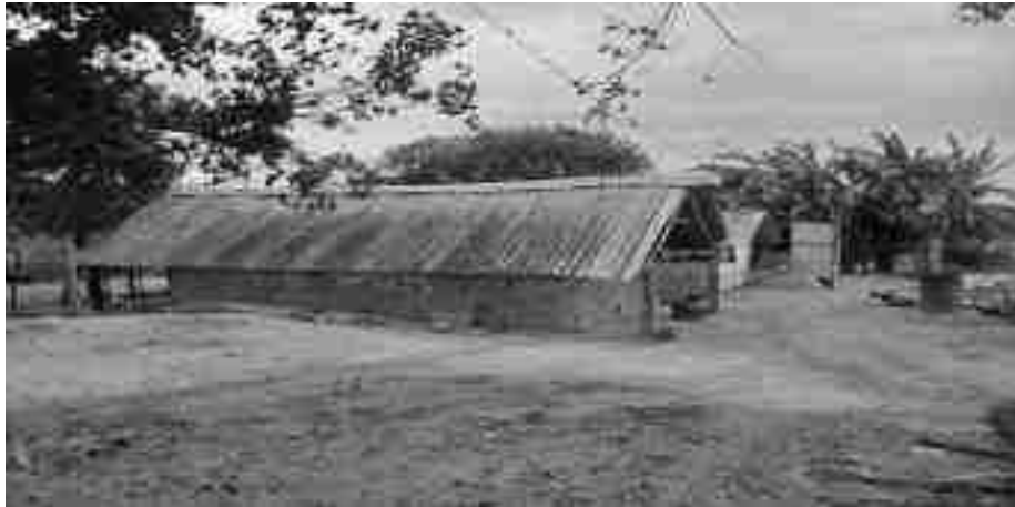
FIG. 14B (Monitoring at the house of Sri Velu Sami, Kattupringiyam Ayyanagar Village)
