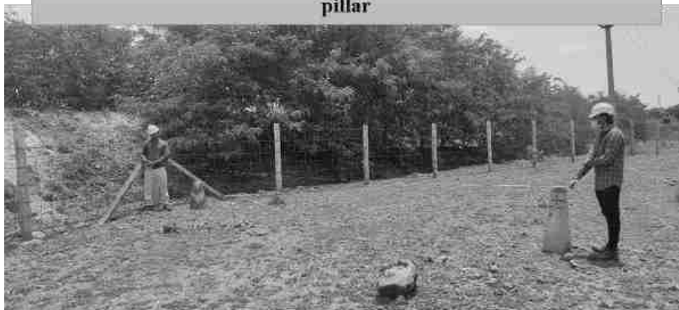
Figure 15. Measurement of wire fencing distance from the lease boundary pillar
