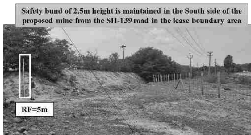
Figure 8. Safety bund of 2.5m height is maintained in the South side of the proposed mine from the SH-139 road in the lease boundary area
