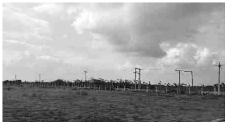
6. Power Line – 50m (NE-SW)
