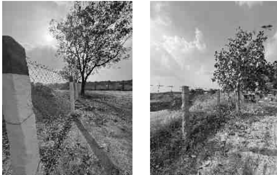
Fencing at Project site
