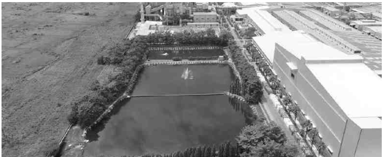
Figure 10-4 Rainwater Harvesting ponds
