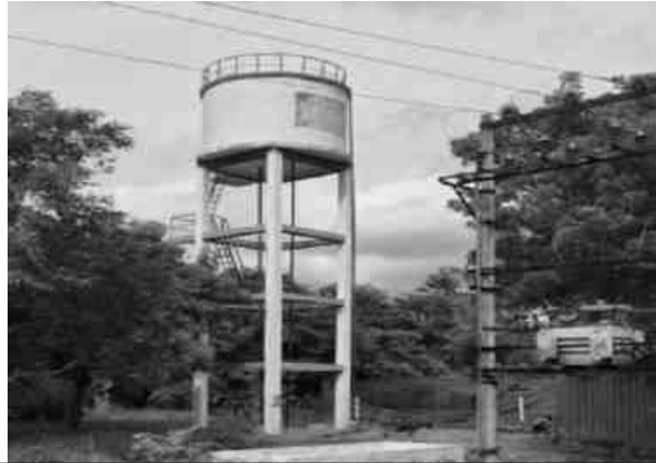
WATER TANK - PAZHAVERI
