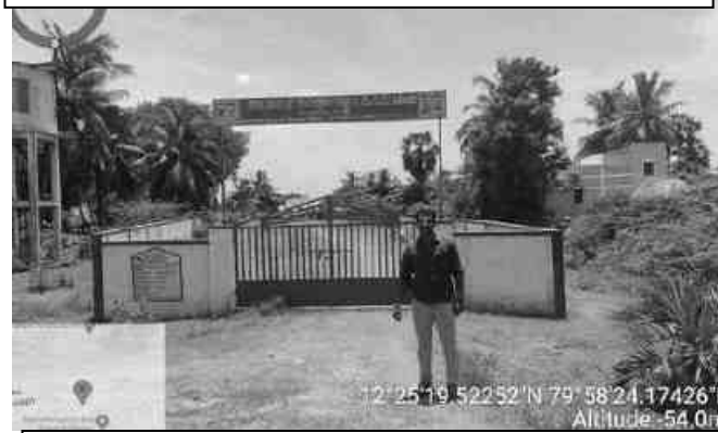
ALAMPATTU VILLAGE, PRIMARY SCHOOL
