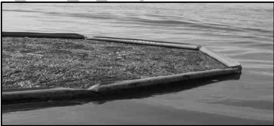
FIGURE 5.1 - BOOMS CAN BE USED TO CONTROL THE SPREAD OF OIL.
