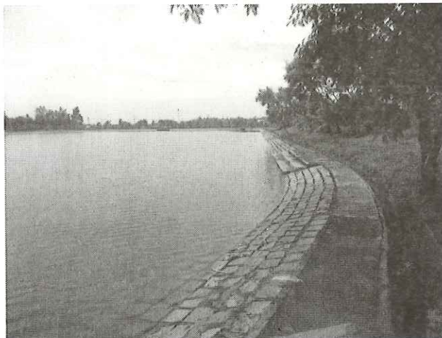
Rain Water Harvesting in Automobile Company, SIPCOT, Irungattugottai
