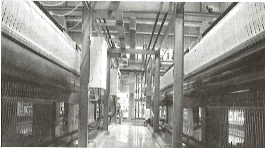
Adoption of Membrane process in caustic soda instead of mercury process as directed by TNPCB
