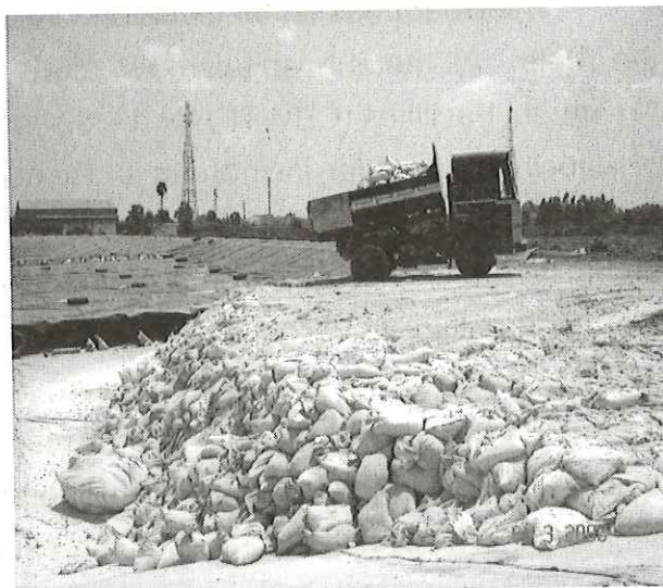
Treatment, Storage and Disposal Facility (TSDF) Gummidipoondi - Landfill
