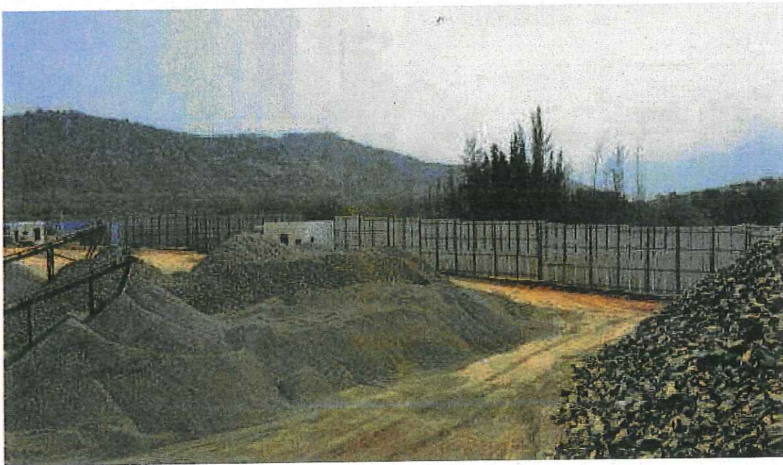
G.I Sheets barrier of 20 feet height on Southern side (inside view)
