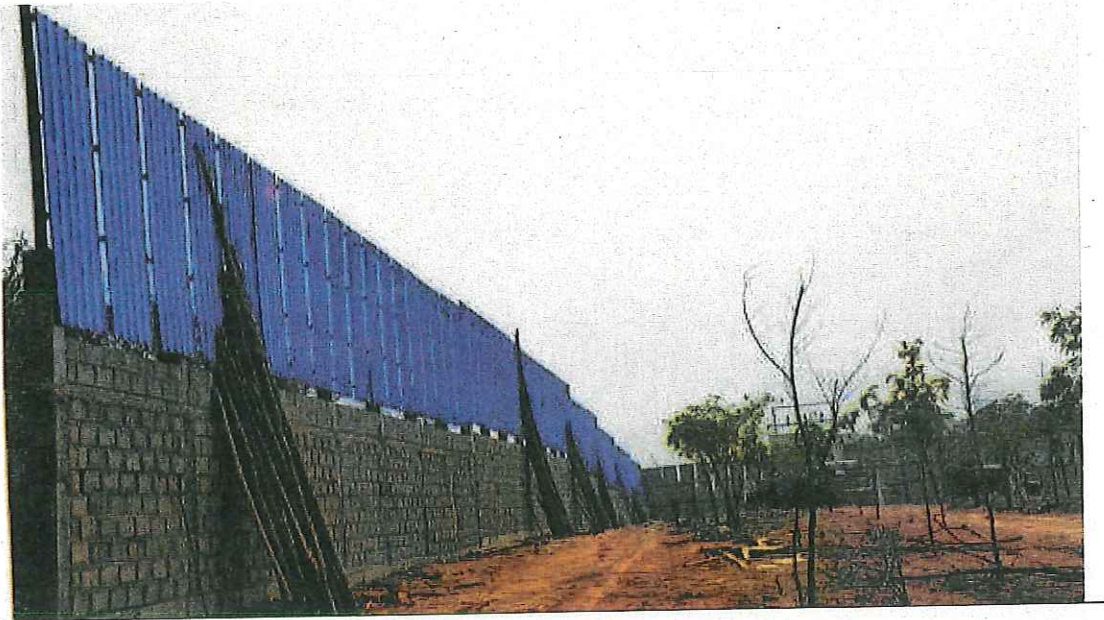
G.I sheet barrier of 10 feet height on Eastern side
