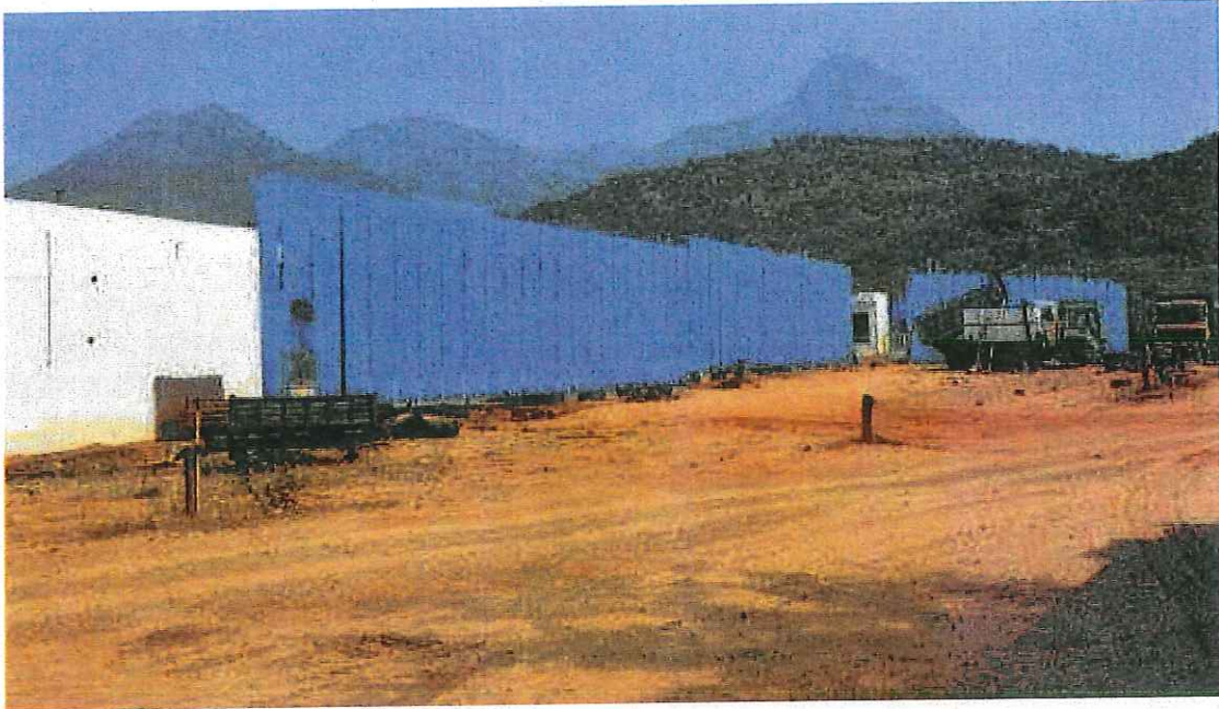
G.I Sheets barrier of 20 feet height on Southern side (Outside view)
