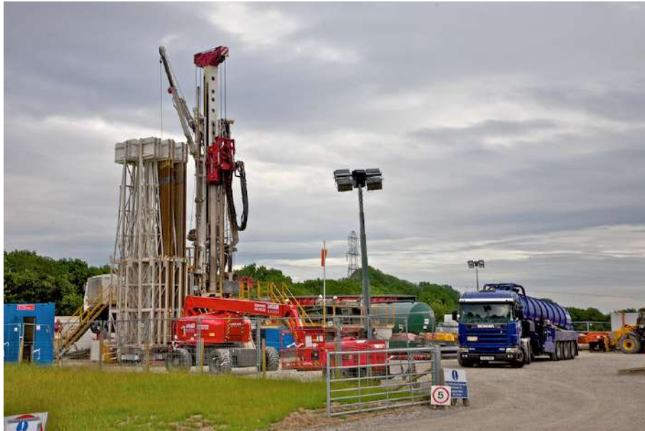
Figure 6 Picture showing a CBM Extraction site
