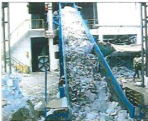
Fig. 2.3 Conveyor towards Pulper
