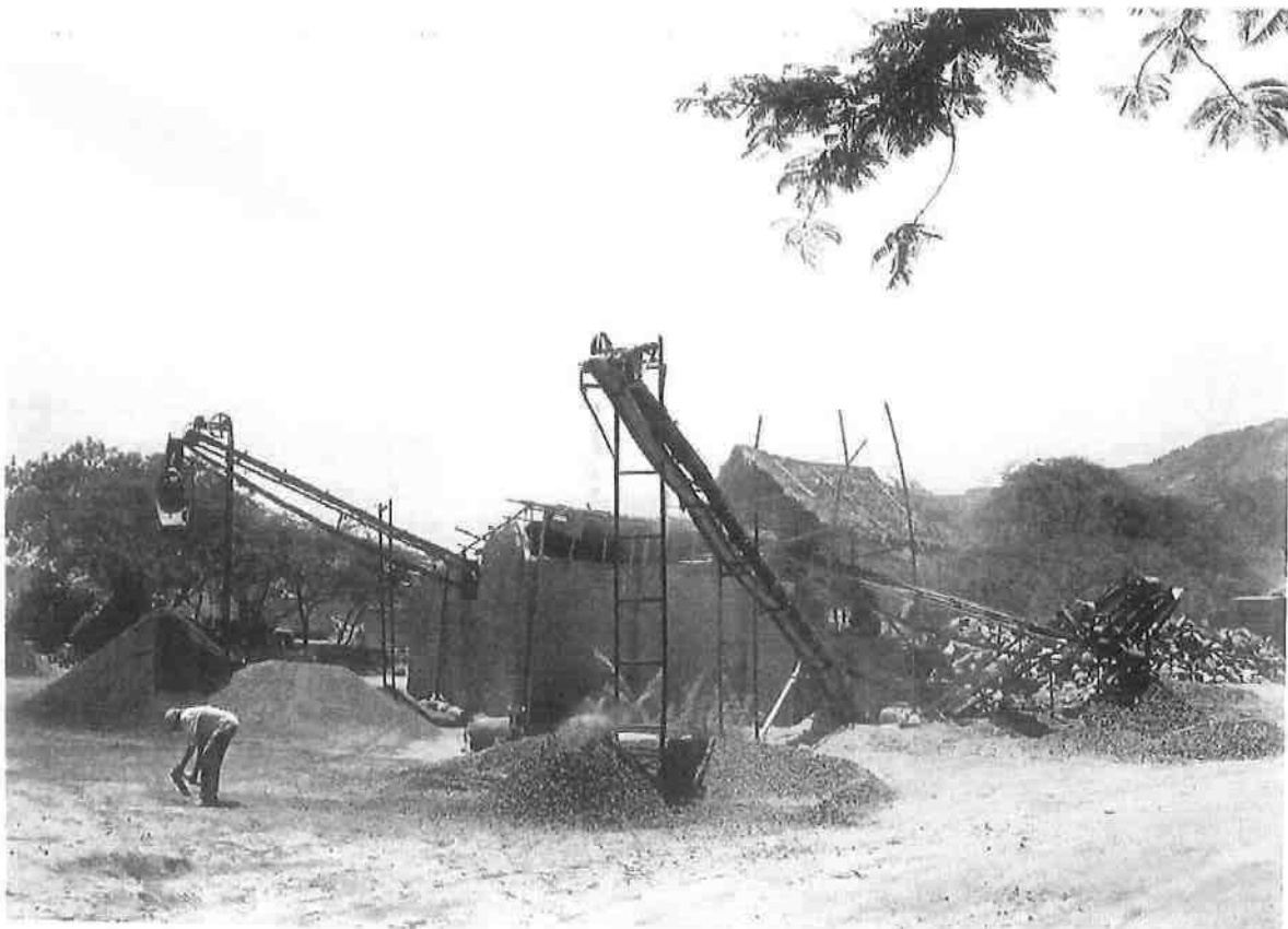
Plate No. 1.3 A View of Stone Crusher in Operation
