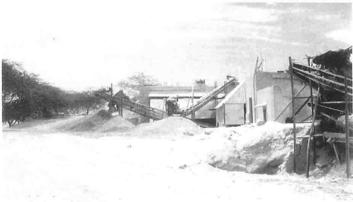
Plate No. 1.4 A View of Stone Crusher in Operation
