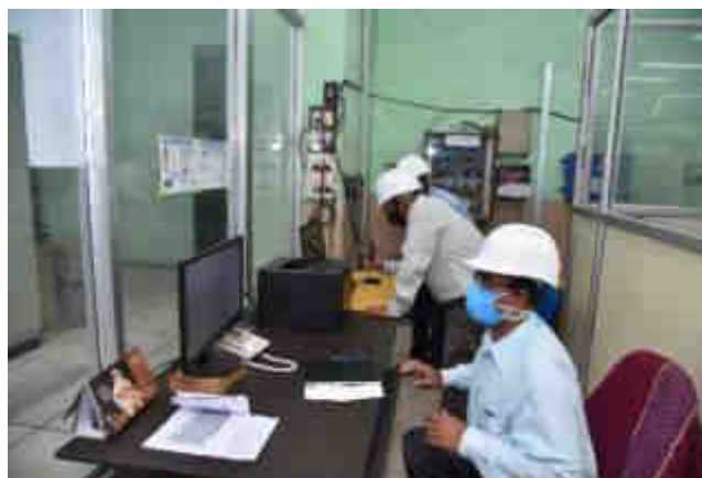
Figure 1 Online data center
