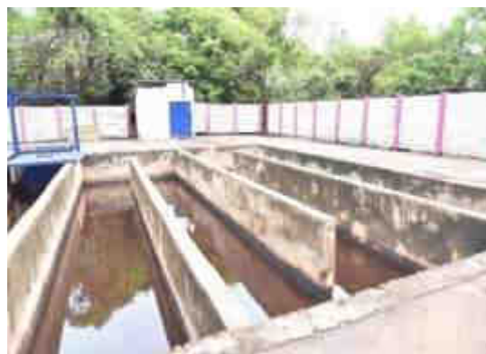
Figure 9 Settling tank
