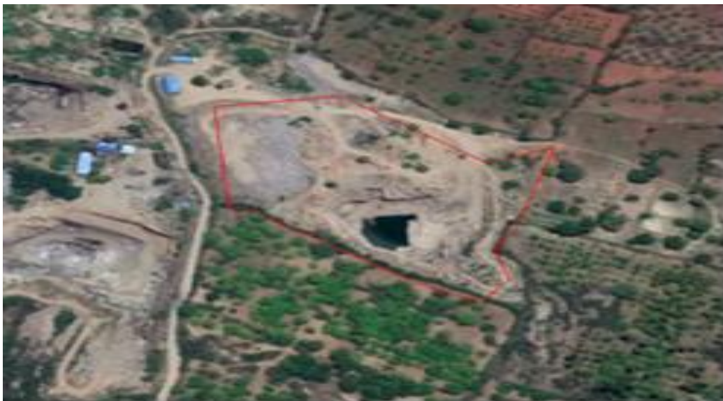
Figure 2: Google Image of the Project Site
