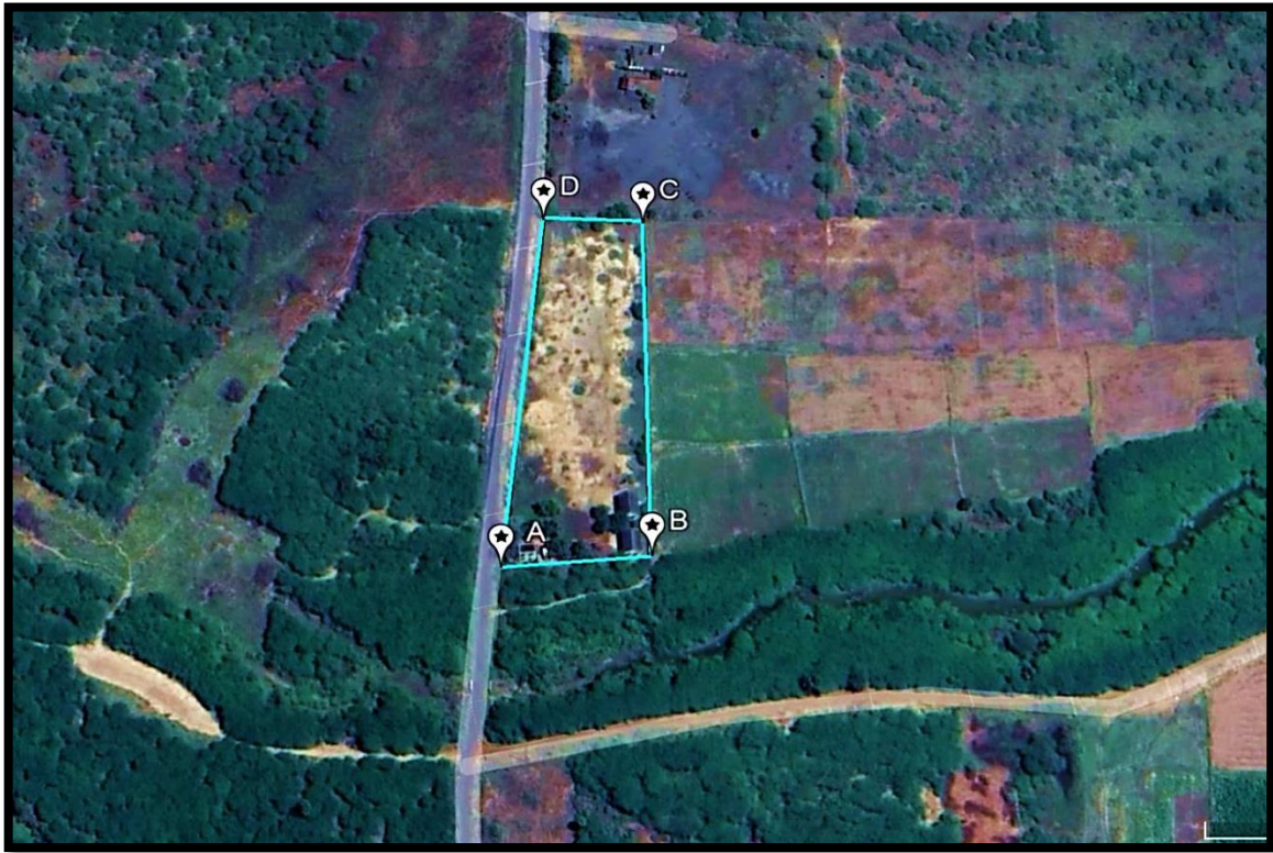
Satellite Imagery of the Project Site
