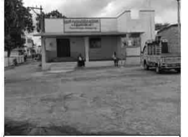
Community Hall, Ramalingapuram
