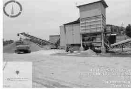
S6 – Crusher Unit (280m, NE)
