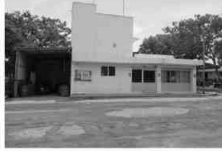
S2 – Crusher Office Room (190m, W)
