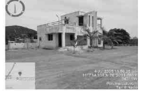
S4 – Crusher Office Room (230m, N)
