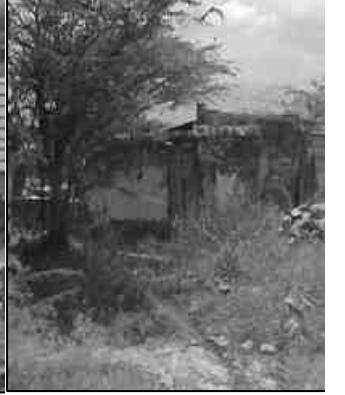
S4- Abandoned Structure - 122m (SE)
