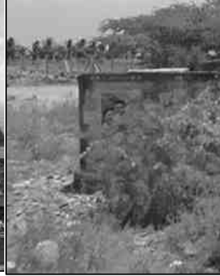
S2-Abandoned Structure - 103m (SE)
