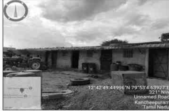
S1 - Storage Shed - 50 m(S)
