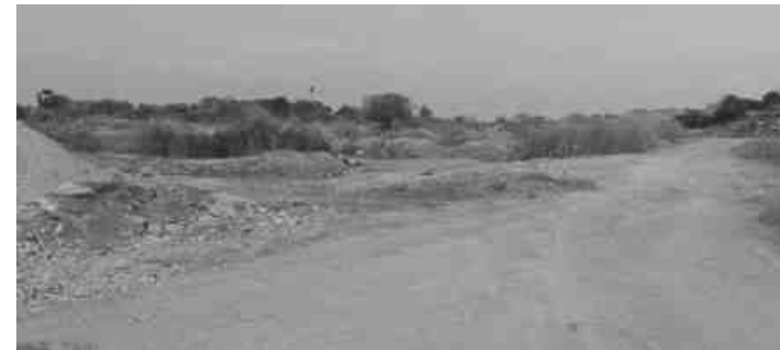
P3 – Thiru. M.Karuppaiya Project Site
