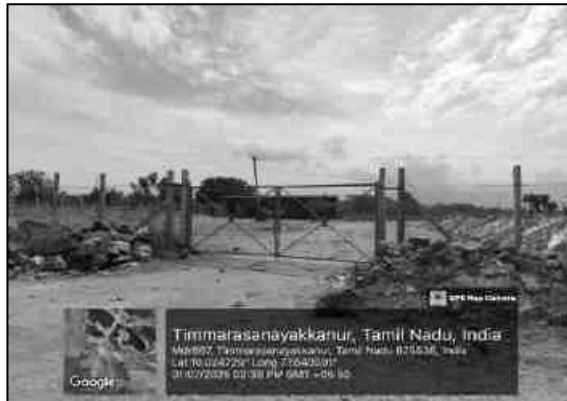
S3- Labourer's Shed - 210m (SE)
