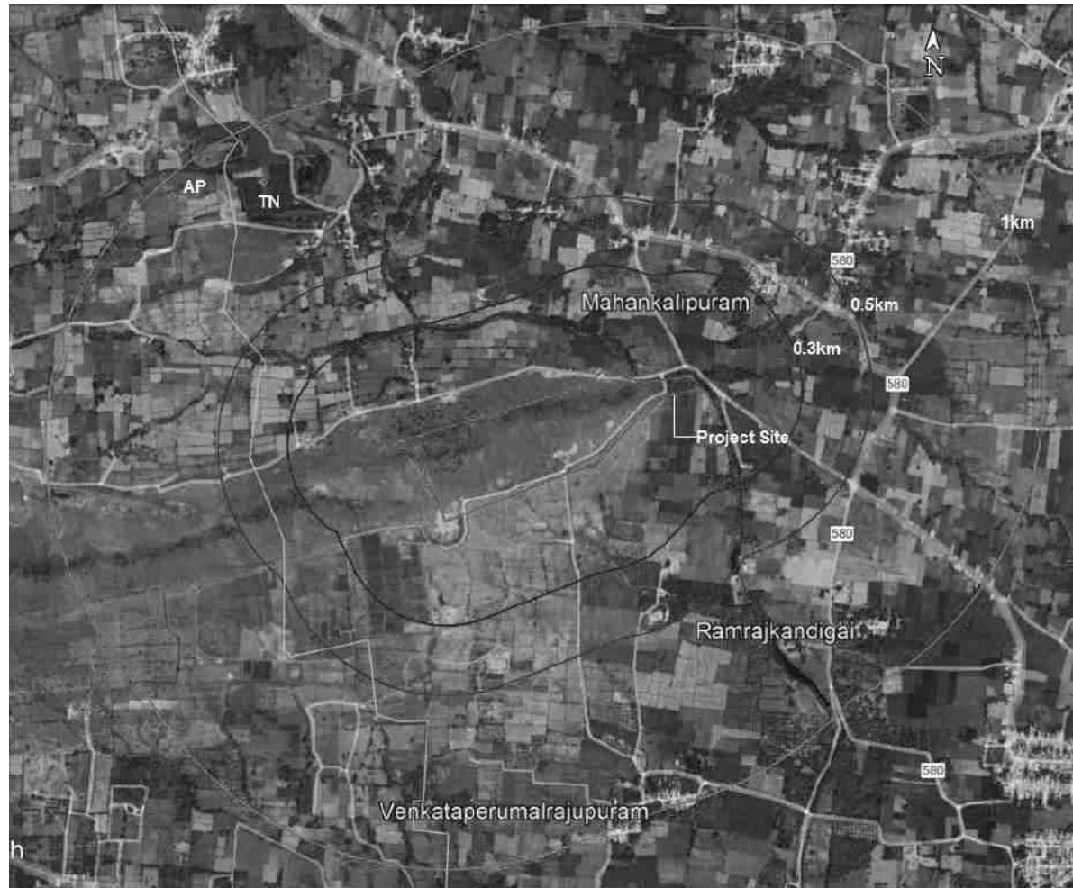
Figure 2-4 Google Imagery of 1 km radius of the lease area
