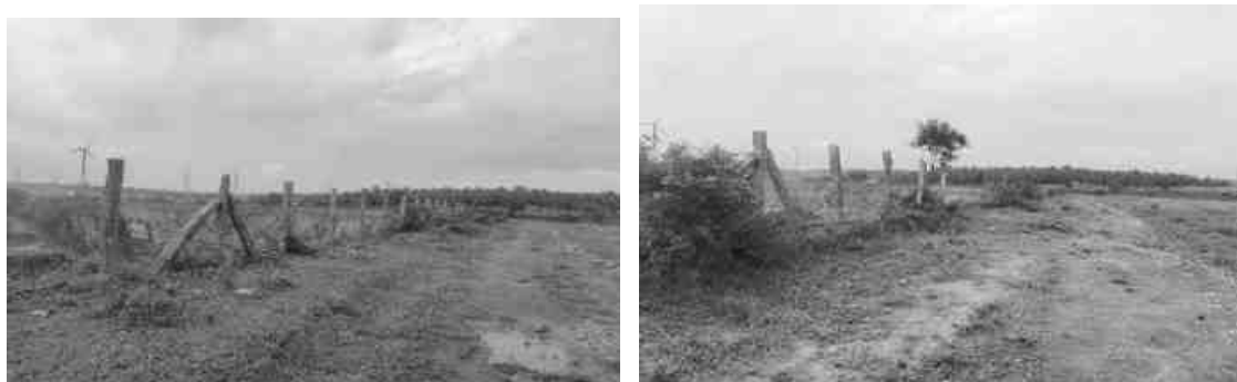
FIGURE 2.2: PHOTOGRAPHS OF FENCING & GREEN BELT
