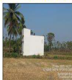
S7- Motor Room- 221m (SW)
