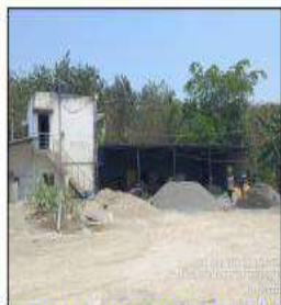
S1- Building Materials Shed- 96m (W)
