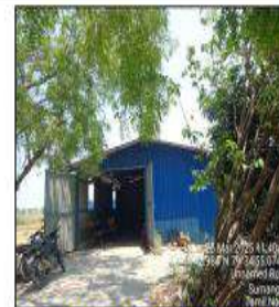
S4- Labourer's Shed- 127m (SW)
