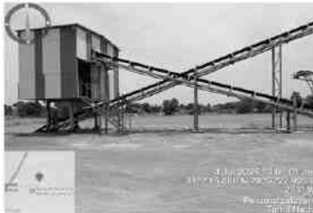
S5 – Crusher Unit (240m, N)
