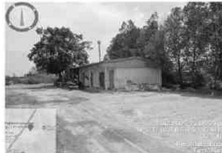
S7 – Worked Shed (265m, NE)
