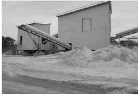
S1 – Crusher Unit (72m, W)
