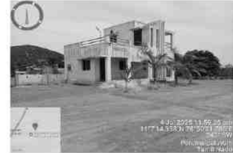
S4 – Crusher Office Room (230m, N)
