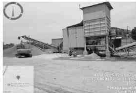
S6 – Crusher Unit (280m, NE)
