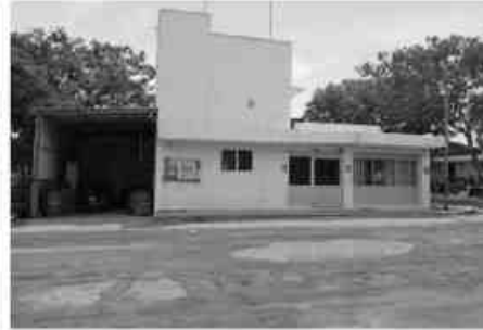
S2 – Crusher Office Room (190m, W)
