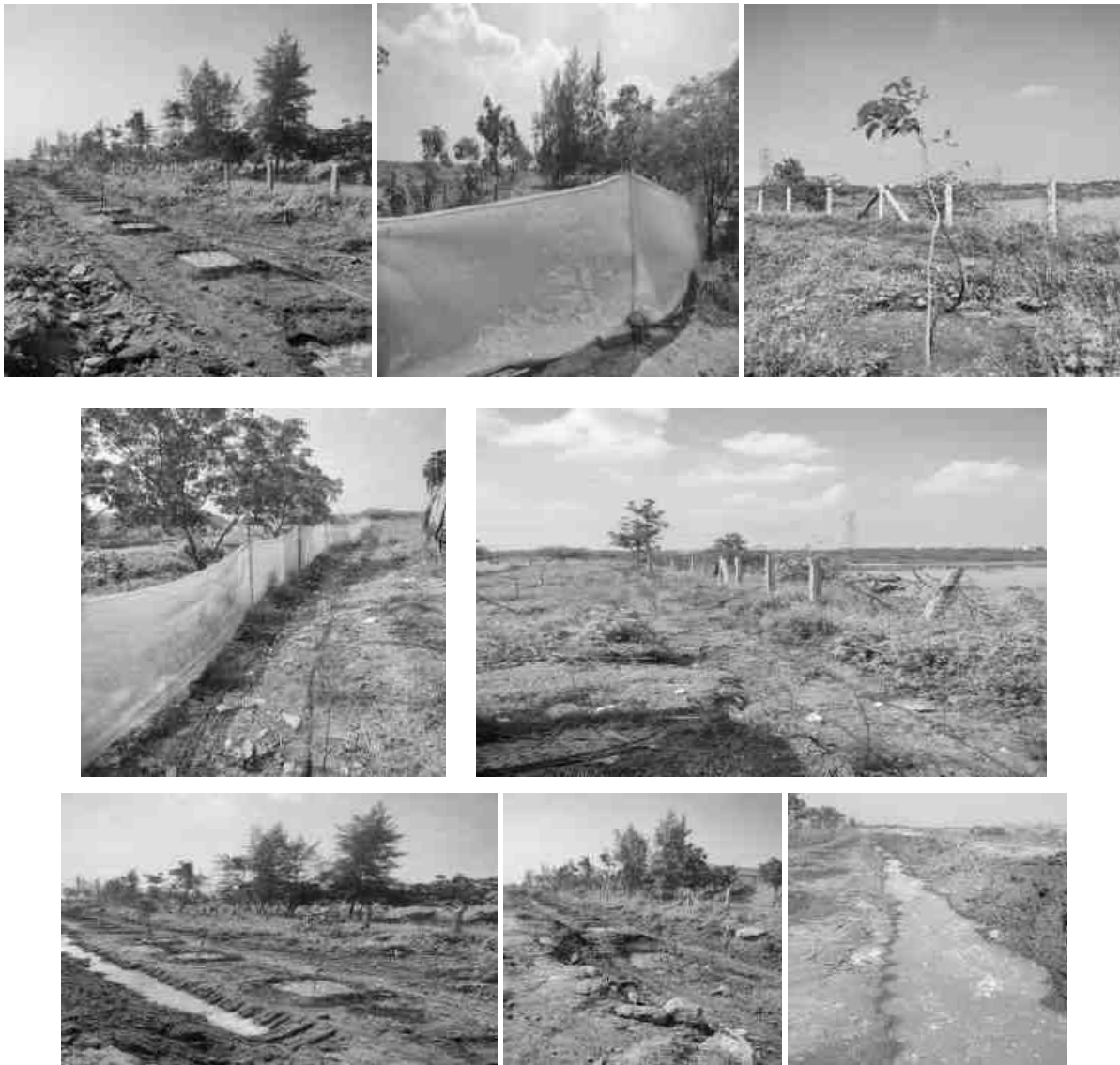
FIGURE 2.1-A: FENCING, GARLAND DRAIN AND GREEN BELT PHOTOGRAPHS
