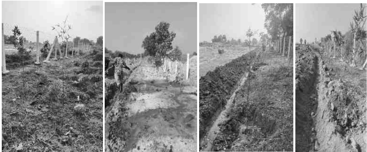
FIGURE 2.2: PHOTOGRAPHS OF GREENBELT & FENCING
