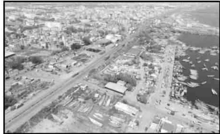
Southern Lower-Level Wharf for FRP Boats
