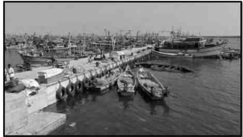
Northern breakwater wharf for MFBs, non-landing wharf
