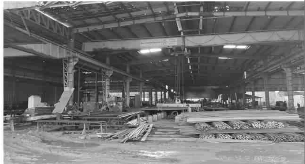
Figure 2-9 Project Site Photographs
