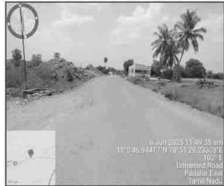
Thiranipalayam Village Road- 10m (S)
