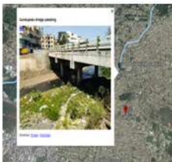
Gundupodu Bridge - 11°39'03.2"N 78°09'26.0"E
