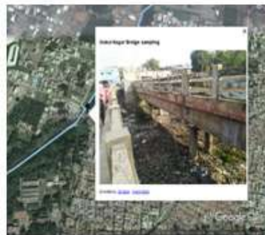
Gokul Nagar Bridge - 11°39'59.0"N 78°10'20.6"E
