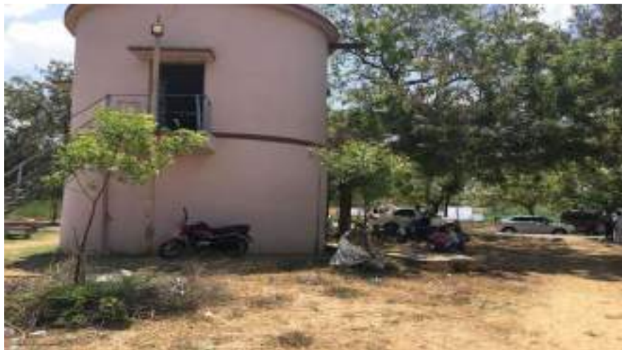
M/s. The India Cements Limited pumping station in River Tamirabharani at Anandakrishnapuram village
