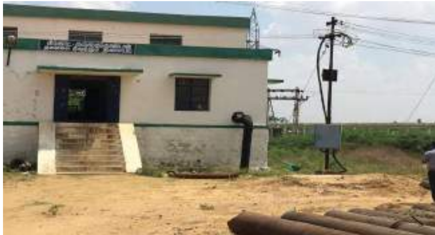
SIPCOT pumping station in the River Tamirabharani at Seevalaperi Village
