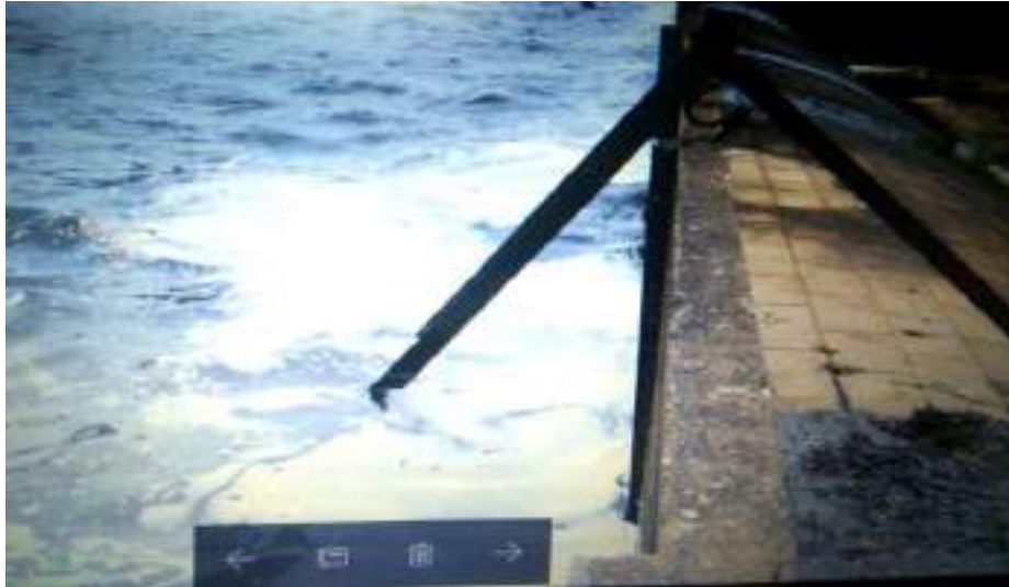
M/s. Madura Coats Limited, Water draw source at Papanasam lower dam
