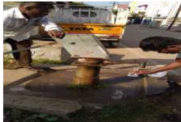
Sindhupondurai Bore well (Sewage Confluence point)
