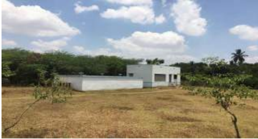
M/s. Arjun pulp and paper India private limited pumping station in River Tamirabharani at Kodaganallur Village
