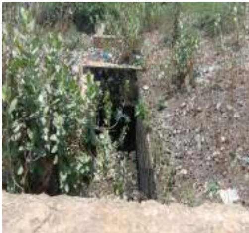
Location: Eral GPRS: N 08° 37' 21.90" E 078° 01' 31.58"
