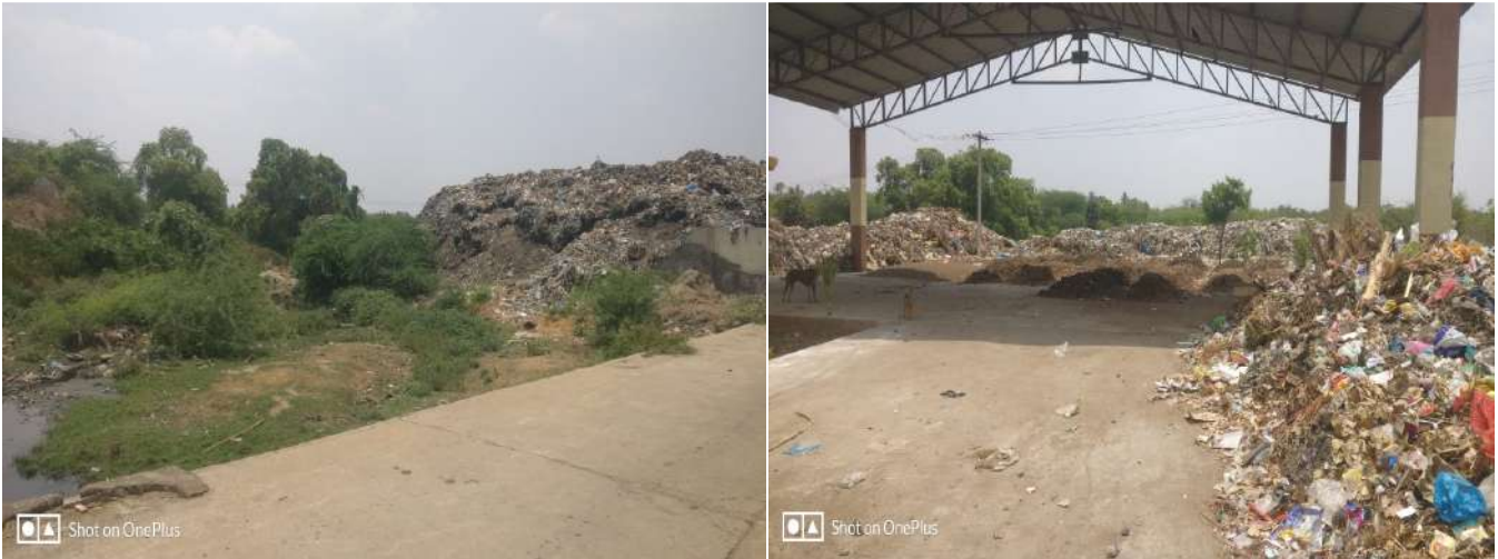
Existing Scenario of the Omalur Town Panchayat Composting unit
