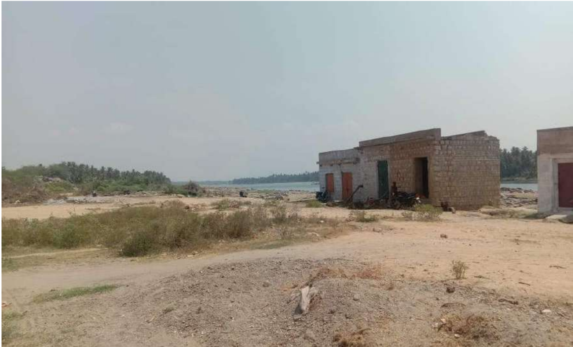
Figure - Downstream of Solasiramani barrage
