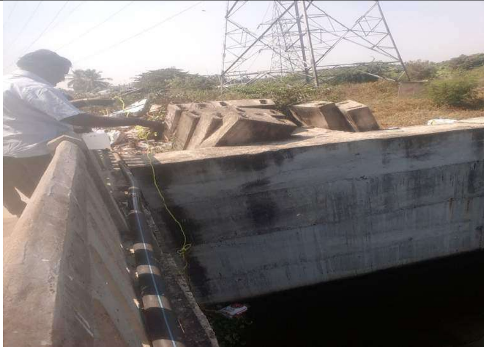
Sampling point at Vendipalayam Barrage at D/s of confluence point of Perumpallam Odai in Cauvery River (No.4)(11°19'52.50"N, 77°45'27.80"E)
