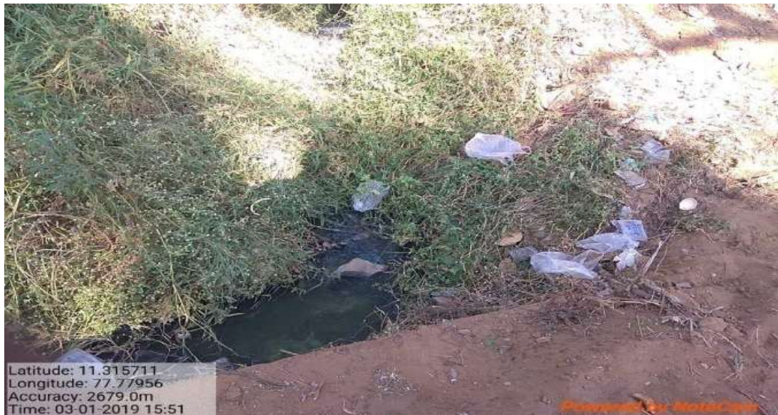
Kokkarayanpettai (Sewage Drain), near bridge
