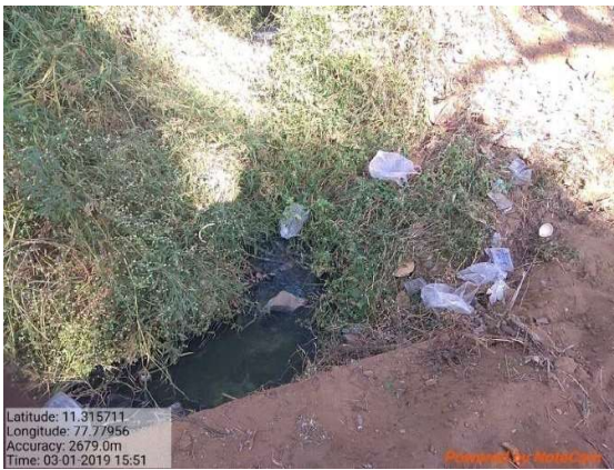
Kokkarayanpettai (Sewage Drain), near bridge
