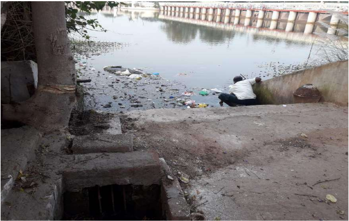
1. Town Sewage drainage outfall, Padithurai, Thirukkattupalli, Thanjavur District.
