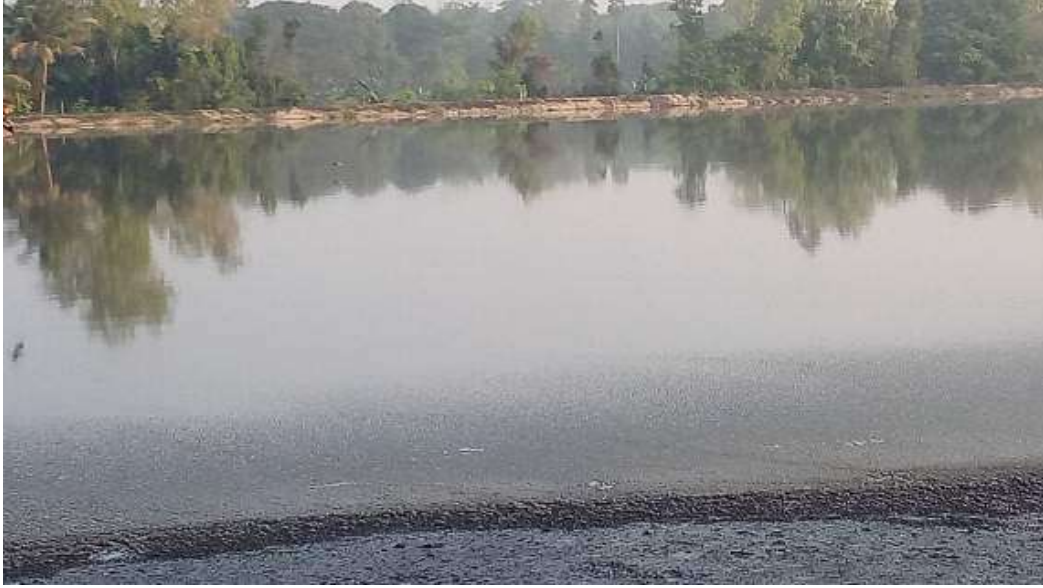
STP Sewage Inlet
