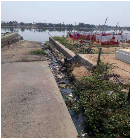
Outfalls near Puthan Santhai, Pallipalayam Municipality, Namakkal District (Map Enclosed - Latitude: 11°22'00" N Longitude:77°44'32" E)
