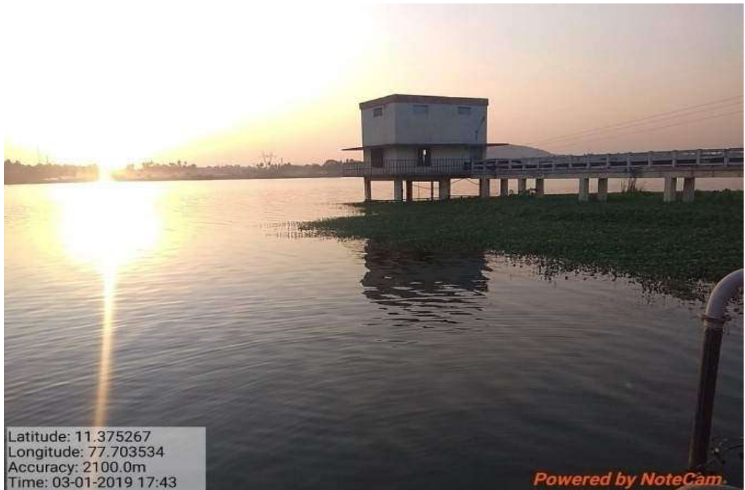
River Cauvery – Seerapalayam near Pumping Station
