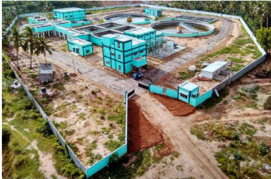
View of the STP established at Vendipalayam by Erode City Municipal Corporation
