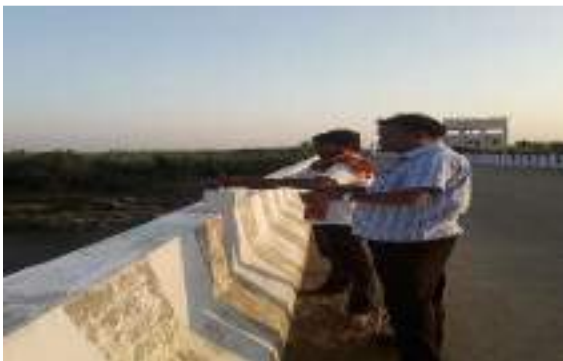
Kallipatti Bridge, Gobichettipalayam
