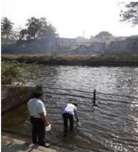
Kalingarayan Canal at River Bhavani
