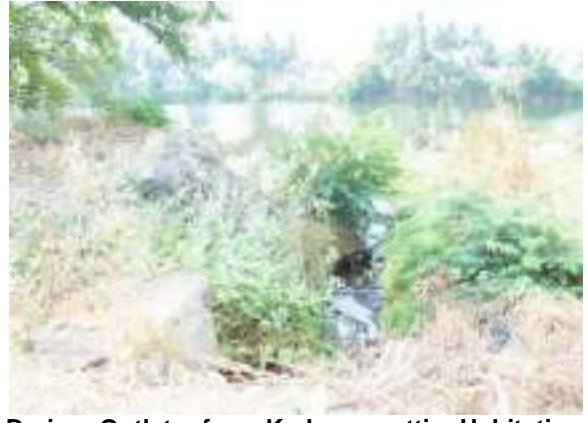
Drain Outlet for Kadayampatti Habitation Kadayampatti Pirivu in Bhavani River H/O Andikulam
