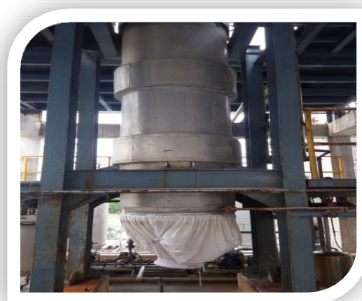
MEE-Vertical Thin Film Dryer
