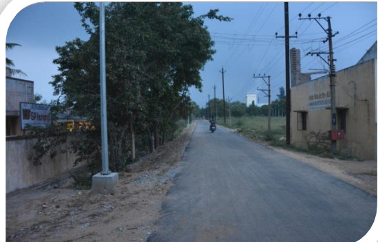
VI Cross Road - After
