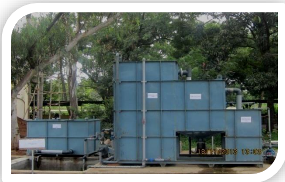
Sewage Treatment Plant
