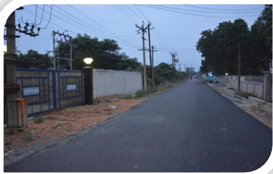
IV Cross Road - After
