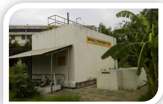
Sewage Treatment Plant – 60KLD
