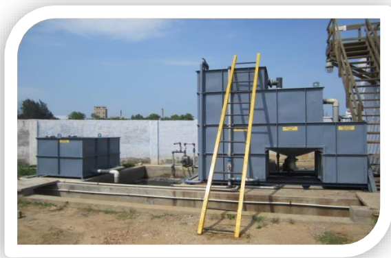
Sewage Treatment Plant
