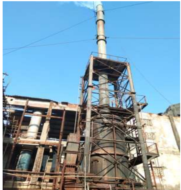
BOILER STACK SPM REMOVAL SYSTEM
