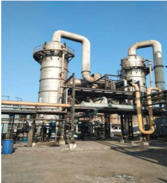
BOILER STACK SPM REMOVAL SYSTEM
