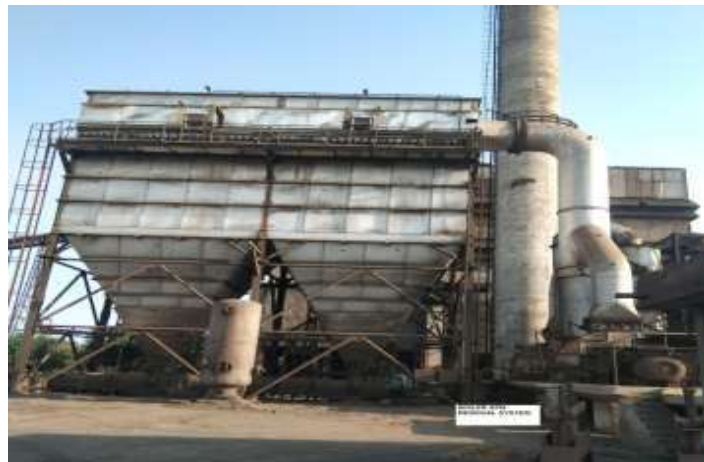
BOILER STACK SPM REMOVAL SYSTEM
