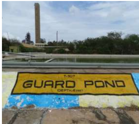
GUARD POND – TREATED EFFLUENT STORAGE
