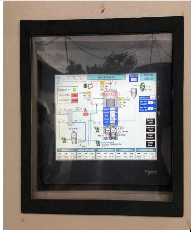
SCADA for MVRE
