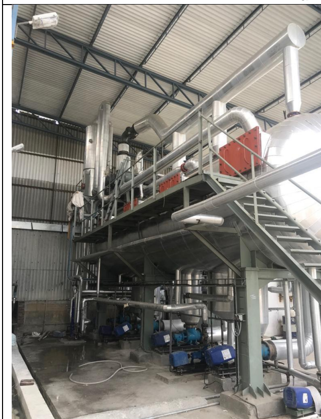
Low Temperature Evaporator installed by the Textile Processing Units
