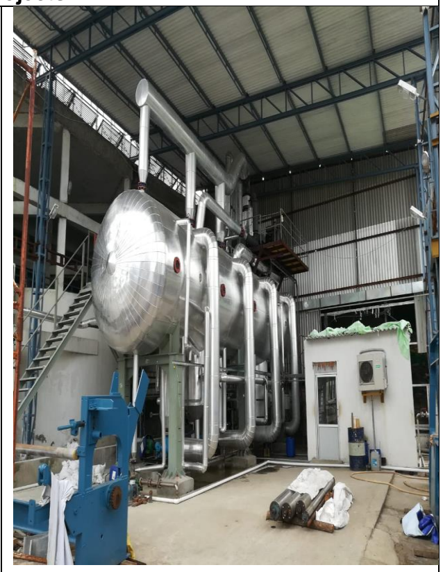
Low Temperature Evaporator installed by the Textile Processing Units
